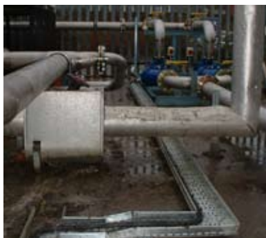
The Free Cooling System on site
