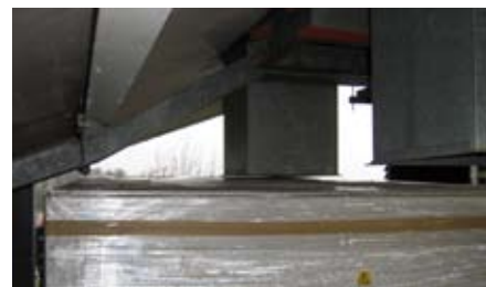
Precision Installation of the new Chillers
