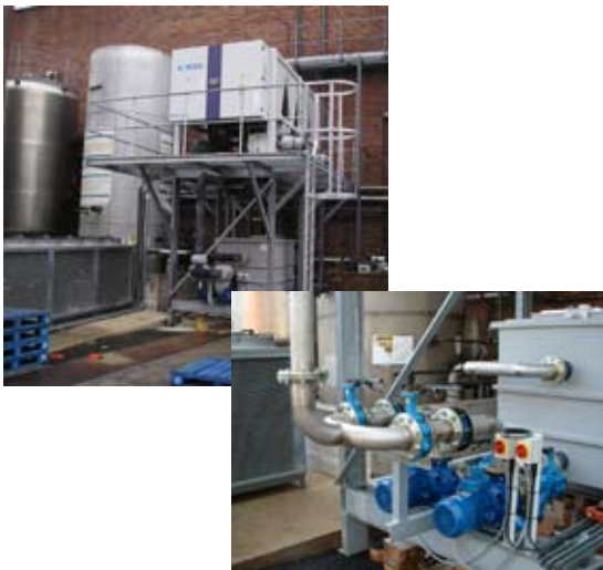
The completed installation
