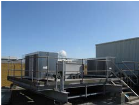
The smooth install of the new units
