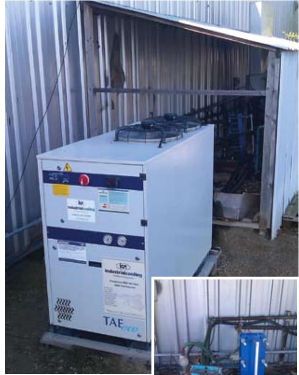
one of the TAE 161 Evo Chiller units and Heat Exchanger supplied by ICS
