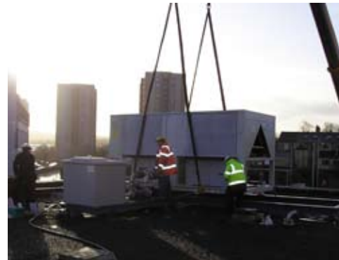
The install on the roof of the Ice Rink
