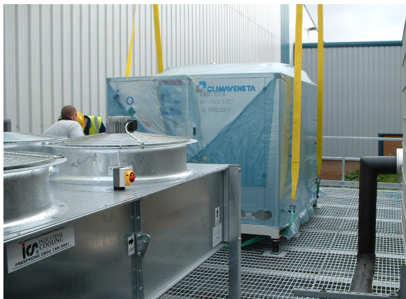
The HRAT FC 0524 unit being installed
